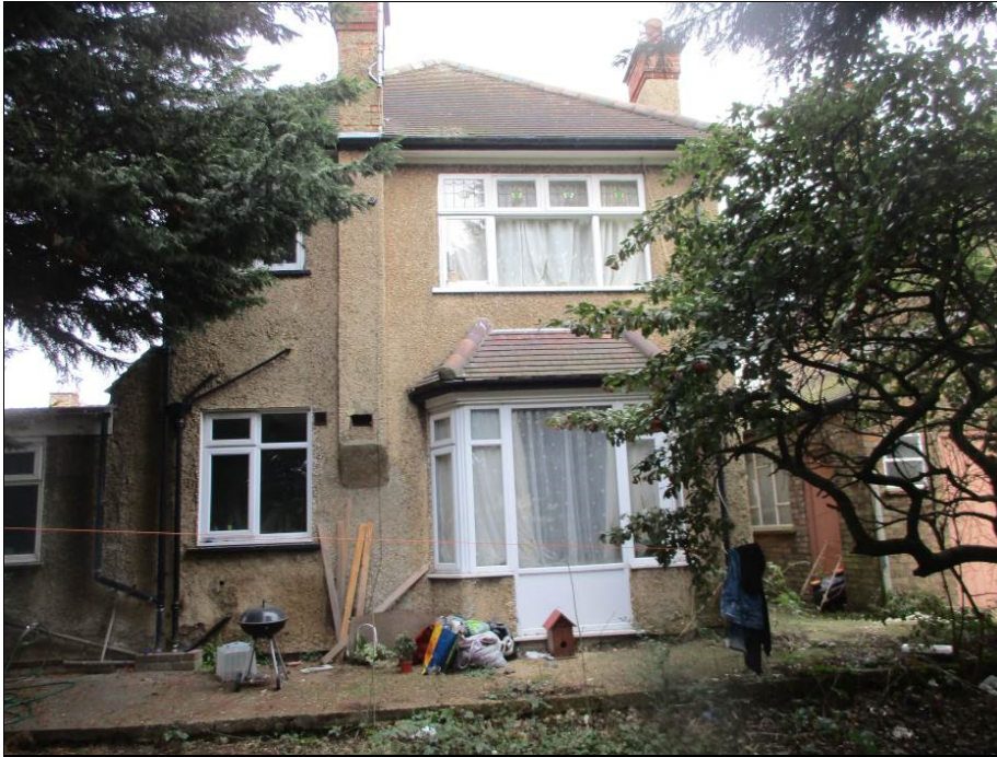
Rear Elevation of no. 9
