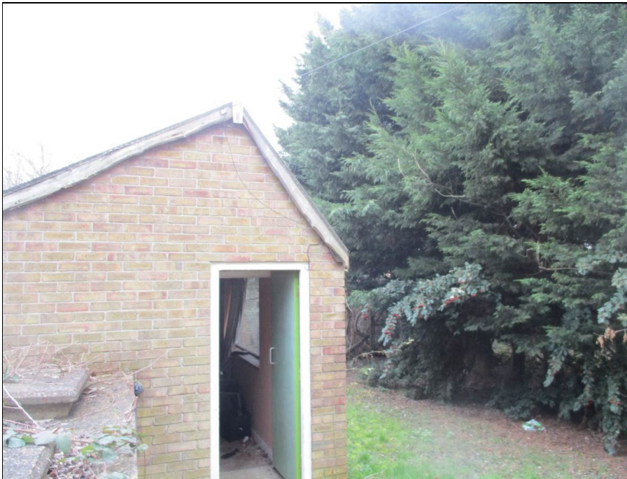
Rear outbuilding at no. 11
