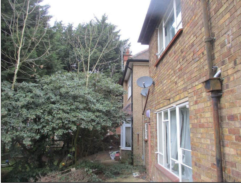
Rear elevations of no. 9 and 11
